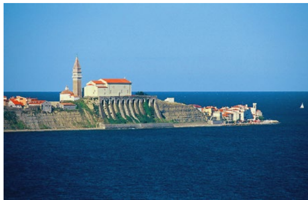
Figure 9: Buttresses below the church in Piran preserved the coastal cliff from natural processes (photo: Matija Zorn)
