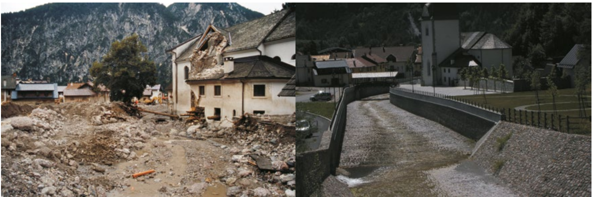
Figure 2. At the end of August 2003, Ugovizza in the Val Canale Valley, Italy, was devastated by a flash flood. Above: the damaged church, which lost its bell tower during the flood. Below: the renovated church and bell tower and the modified riverbed (photo: Matija Zorn).
