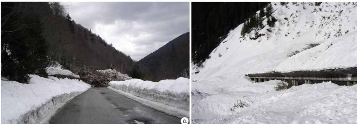
Figure 8. The Transfăgărășan highway (a.) a snow shed (b.) affected by a huge snow avalanche, produced in March, 2005
