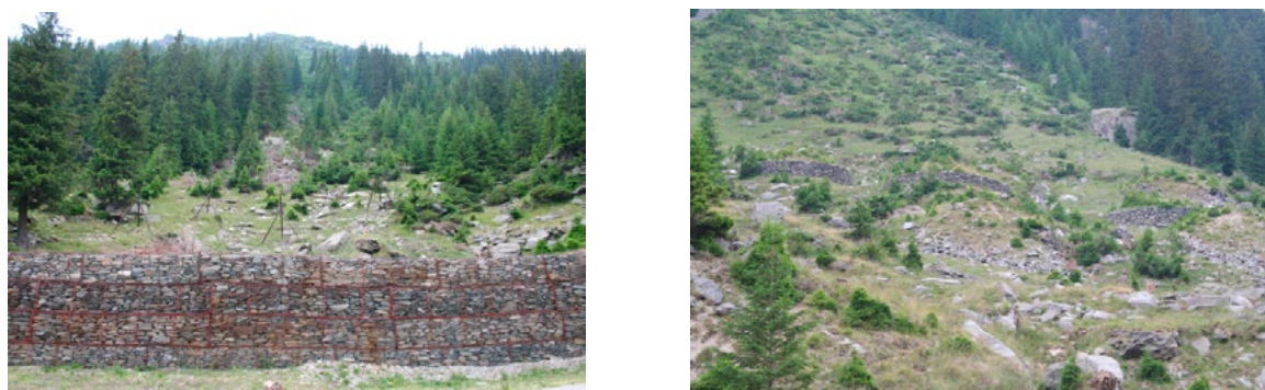
Figure 6. Wooden tripods or avalanche barriers, or deflecting dams made use of in the Capra glacial valley
