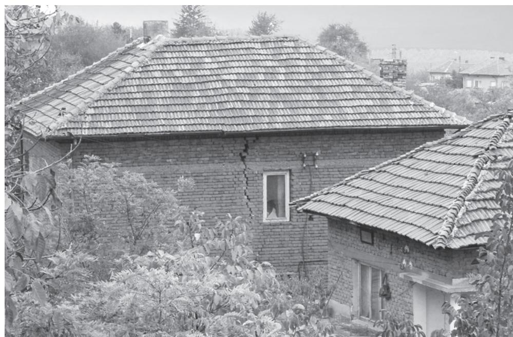
Fig. 5. Cracked house in Somovit village. The concrete slab is cut (21.10.2012)
