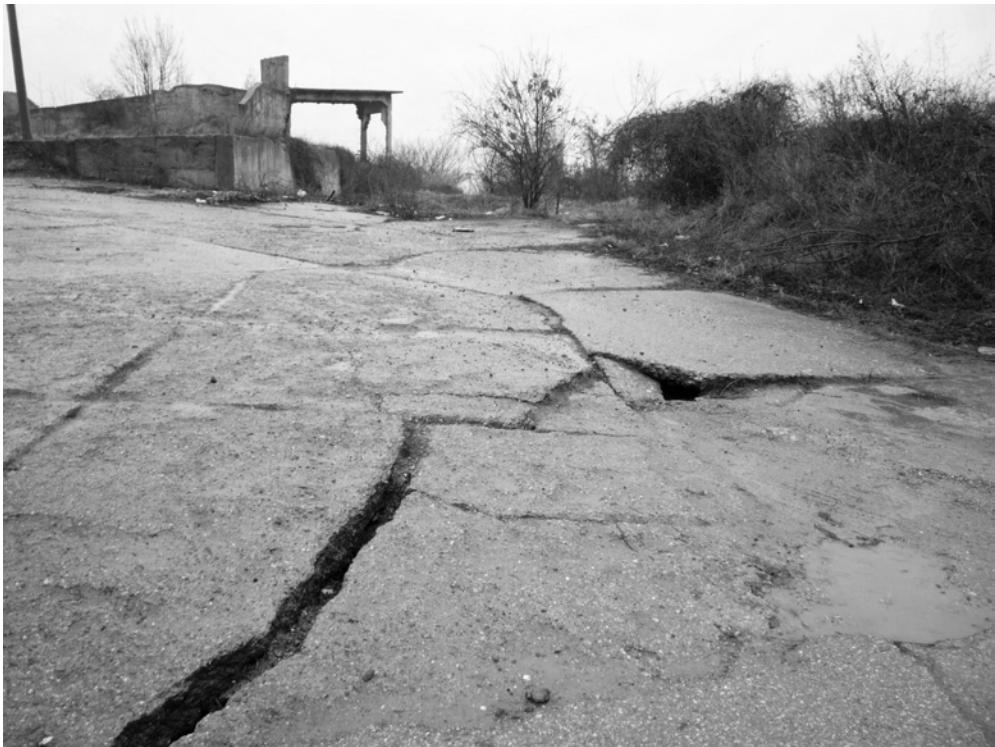
Fig. 4. Deformations on the road at the Center for technical inspection of cars (07.02.2013)
