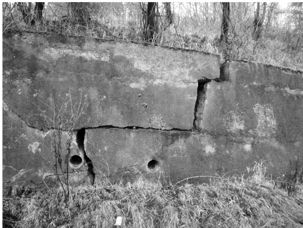
Fig. 3. Retaing wall damaged by landslide movements (22.10.2012)
