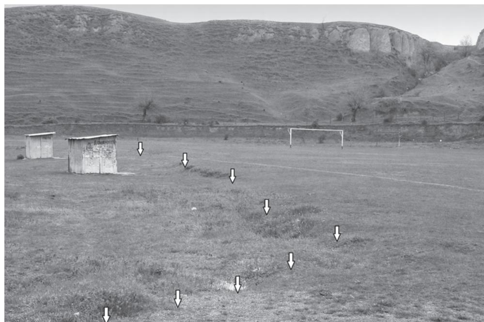
Fig.6. Landslide damages of stadium terrain, "Shipka street" Landslide, Nikopol Town (16.04.2013)
