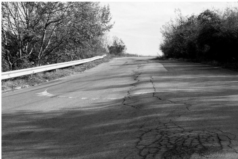
Fig. 2. Deformations affecting the road Lom – Kozloduy (30.10.2013)
